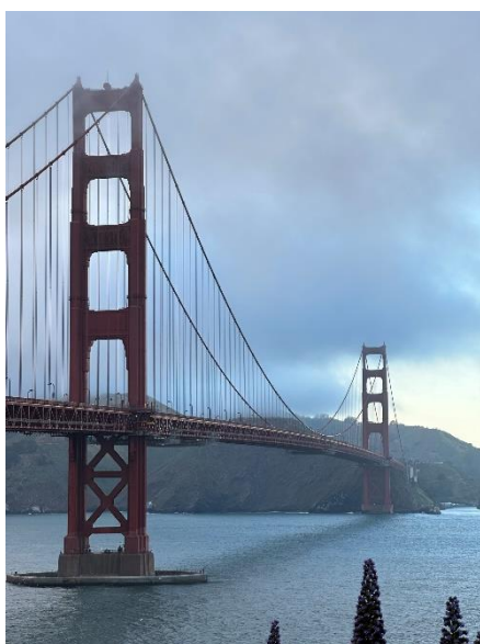
Golden Gate Bridge in San Francisco
